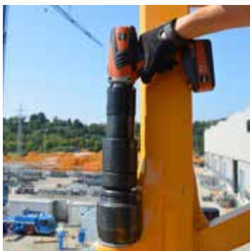
Tower section assembly with battery nut runner
