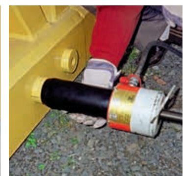
Dismantling of taper pin connection with bolt tensioner
