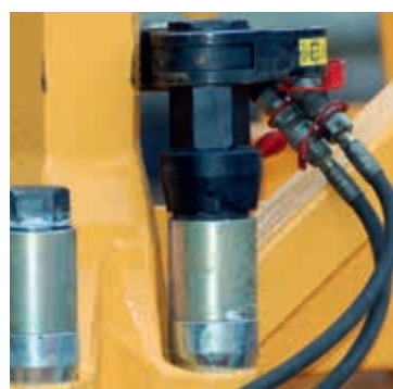
Tower section assembly with FSX
